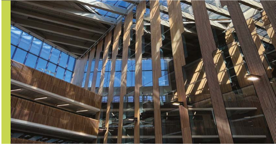
Atrium in Belfast Campus
