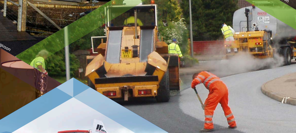
Road laying Inverness by Gordon Douglas
